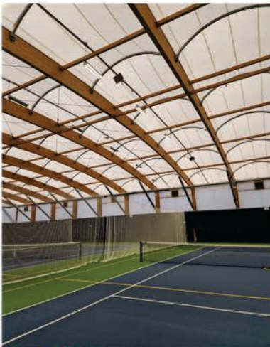
PRECEDENT IMAGE SIMILAR ROOF COVERING SYSTEM
